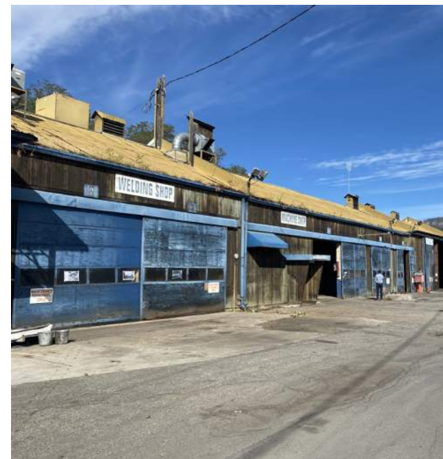
Figure 68. Exterior view of the Machine Shop
