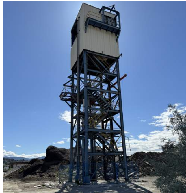
Figure 70. The Chip Tower
