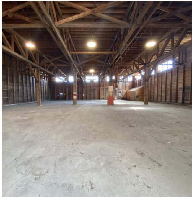
Figure 65. Inside No. 5 Shed
